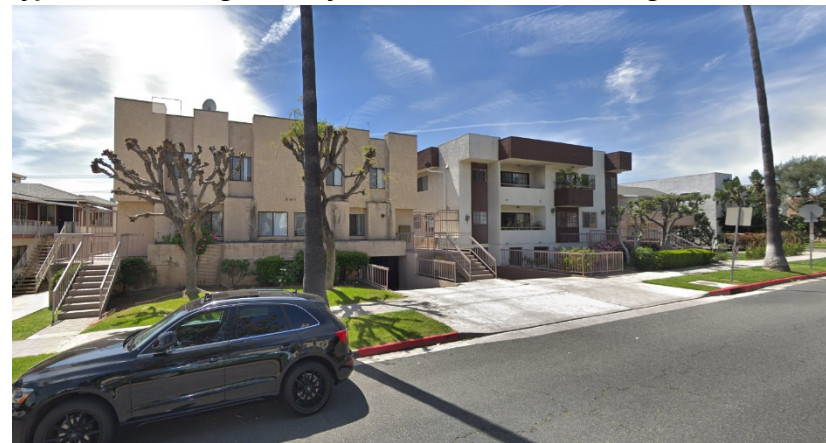
Typical Medium High Density Residential (Glenwood Neighborhood)
