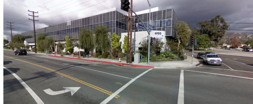
Typical Commercial/Residential Mixed Use (Glenwood Neighborhood)
