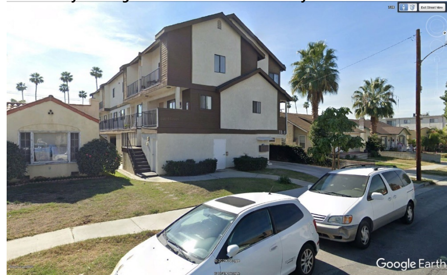
Multi-family building in R-1 Residential Low Density zone
