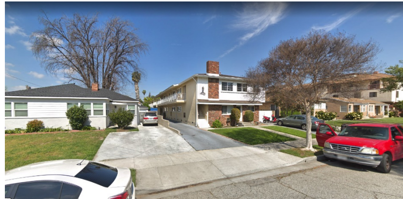
Typical Moderate Density Residential (Riverside Rancho Neighborhood)
